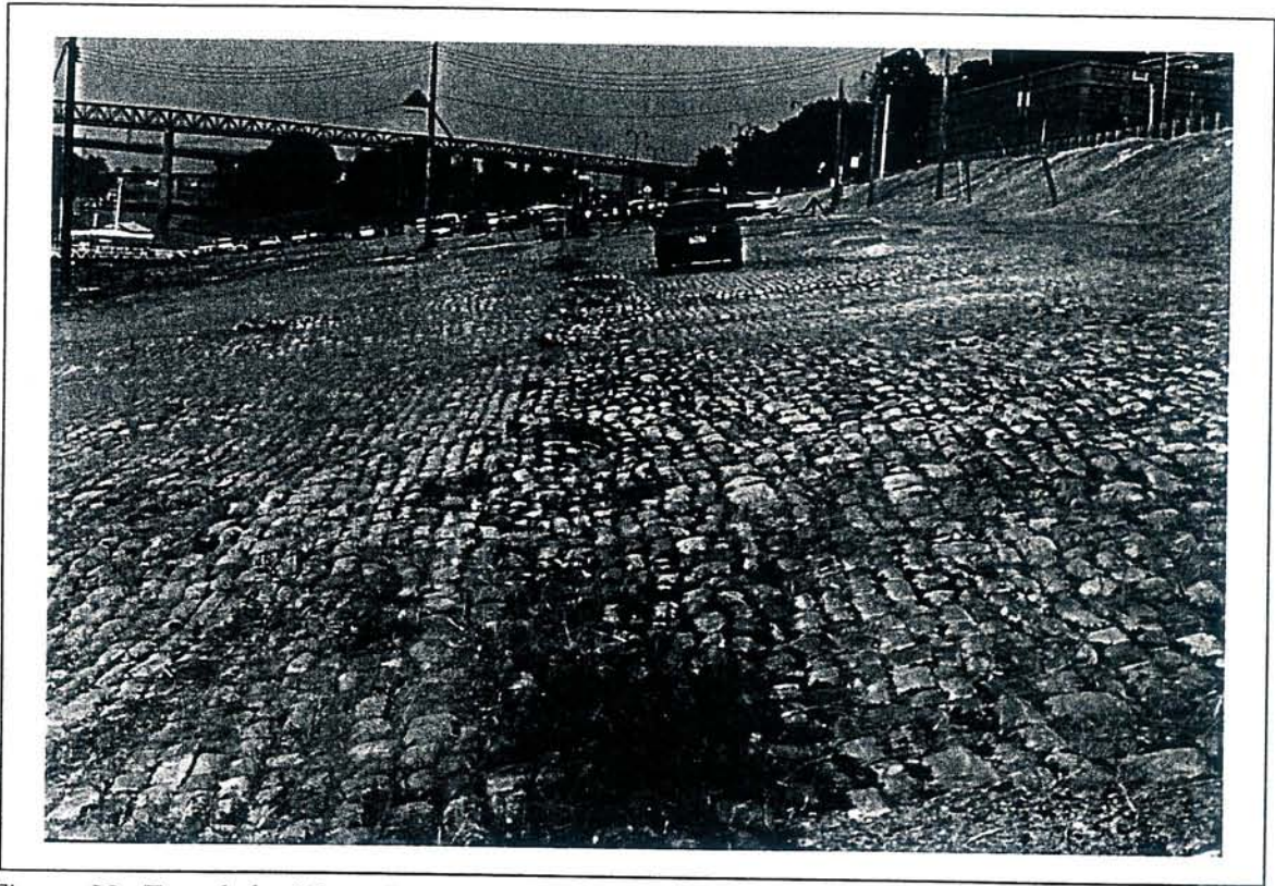
Figure 33. Trench for Water Line (View to the North).
