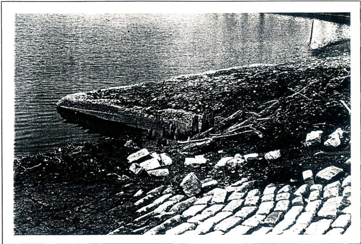
Figure 32. Gayoso Street Sewer (View to the North).
